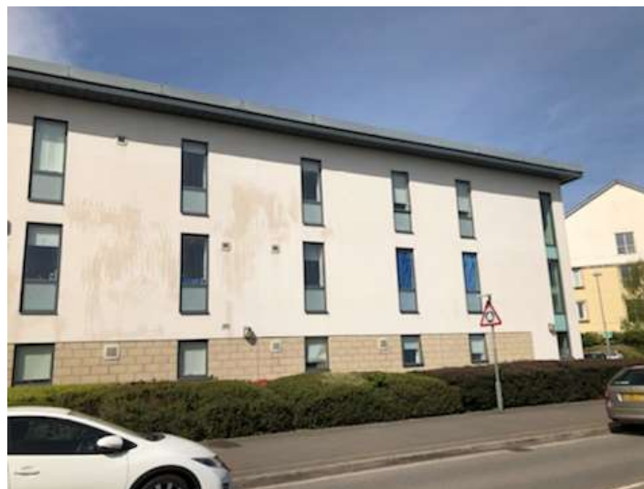
Harbour Rd rendered elevation softwashed
