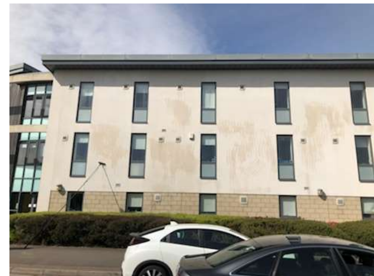
Harbour Rd rendered elevation softwashed
