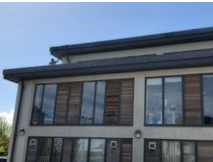
Courtyard / Harbour Road Wing, box gutters cleaned
