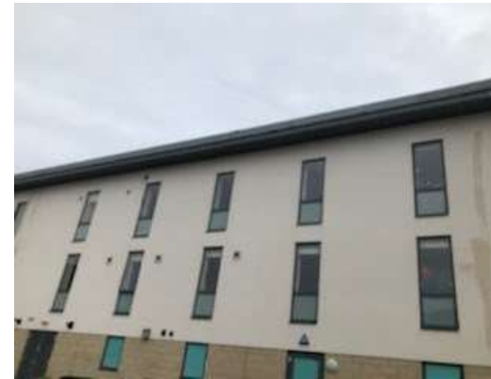
Harbour Rd rendered elevation softwashed
