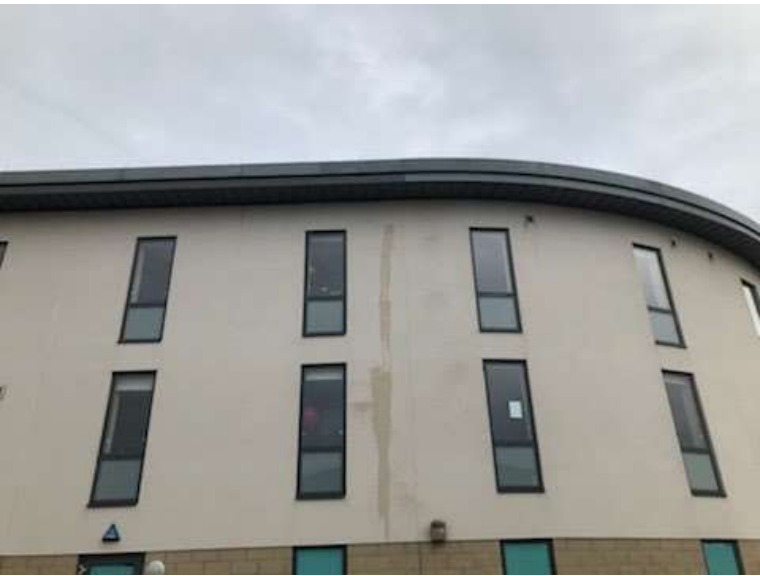
Haven Rd box gutters cleaned
